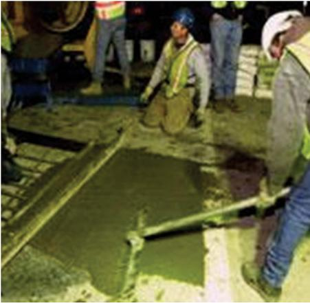
FIGURE 3: Repair of Pennsylvania Turnpike using CBPC-based Monopatch (courtesy: Bindan Corporation, USA).
